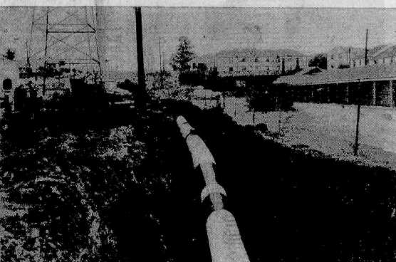
Part of Transcontinental Gas Pipe Line Corporation's 36-inch main-line loop laid on Public Service Electric and Gas Company's transmission right-of-way through the Nutley-Belleville area.
